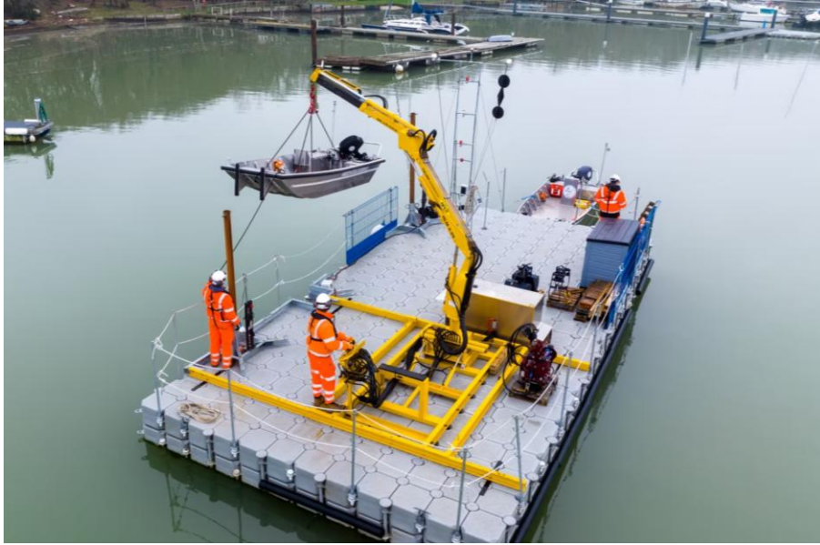
Figure 8. Example 2 Shallow draft work platform / Pontoon system
